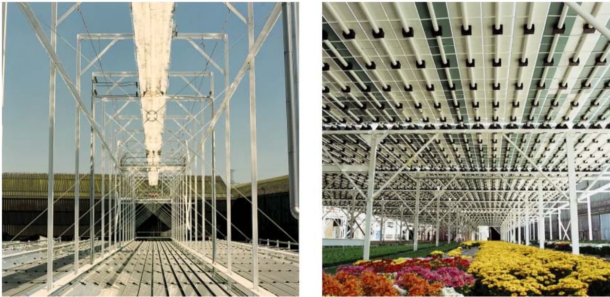
Figure 5.4 Energy production above and horticulture underneath a linear Fresnel collector field
